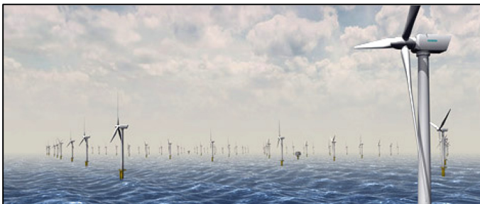
Fig 1. Sheringham Shoal Offshore Wind Farm in United Kingdom
